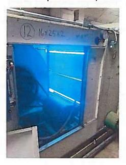
This is a picture of our UV installed in the ductwork. Essentially all of the air gets sucked out of the classrooms, passes through these UV bulbs to kill pathogens and then is mixed back into the air (combination of fresh/recycled) that goes into classrooms.
